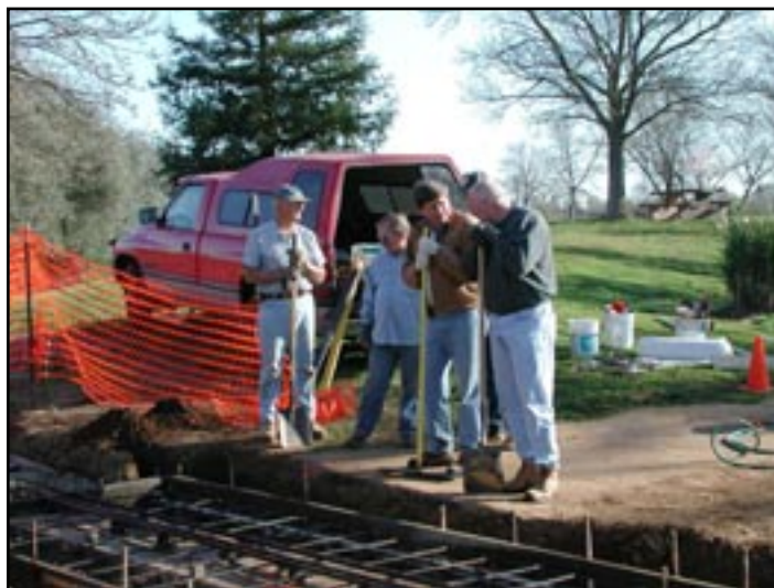
Engineers provide shovel support waiting for concrete.
