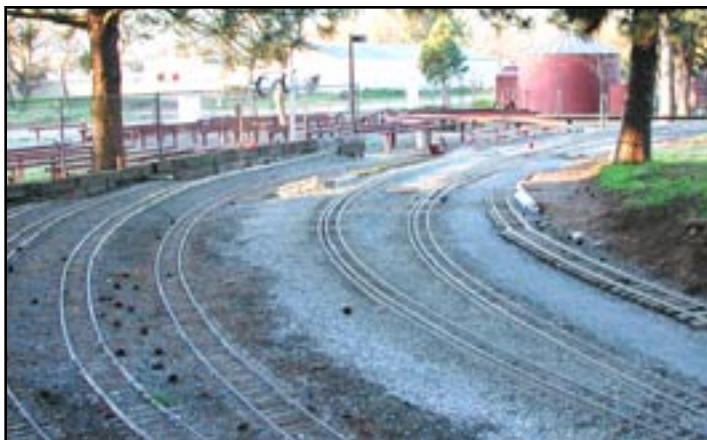
View of new lead tracks and gravel work
