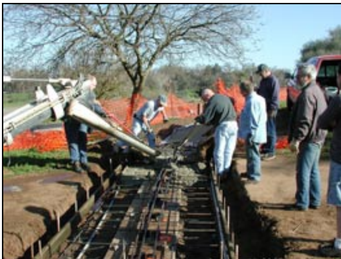
Doing the final concrete pour at Riverview crossing.
