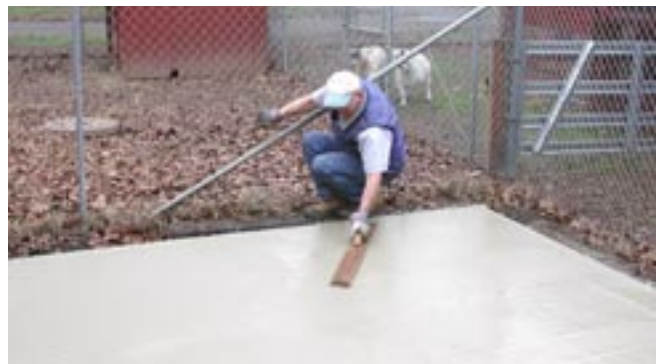
Pete Arney - putting finishing touches on new pad for storage shed.
