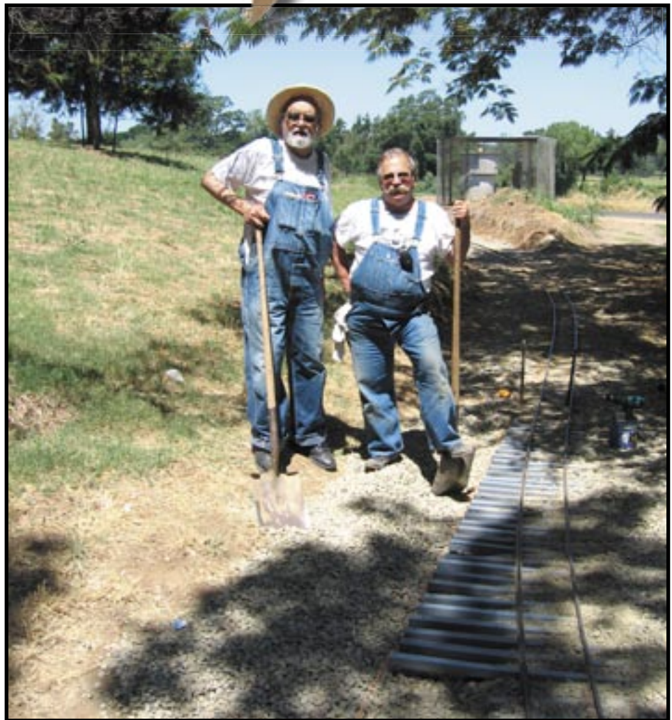
Al Shelley and Karle Mahler on July 7th putting in longer ties for the turnout.
