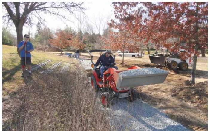
Member Bob Silva from Merced who brought his tractor and helped move ballast. Andrew Sach (on the left) waiting to rake the roadbed before placing track panels.
