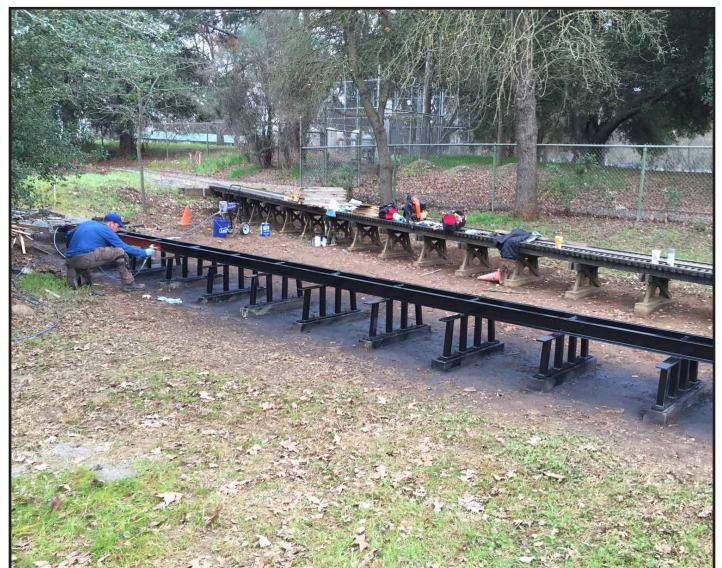
Andy Bechielli painting the trestle - getting this project done.
