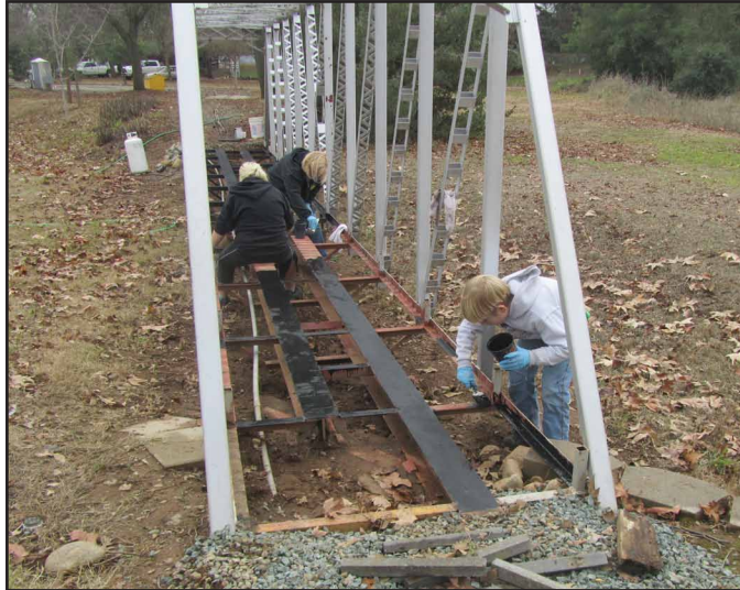
Heidi, Maren and Ryan painting the tops of the girder. Gordon and Andrew installing the guard rails.
