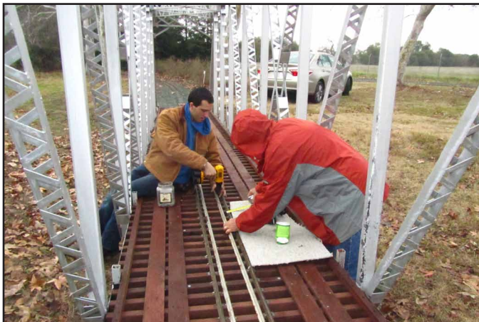
Heidi, Maren and Ryan painting the tops of the girder. Gordon and Andrew installing the guard rails.
