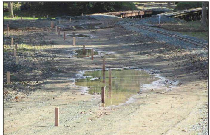
The stakes are the path of the new road bed.
