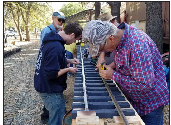
Track panel building for the inside loop project.
