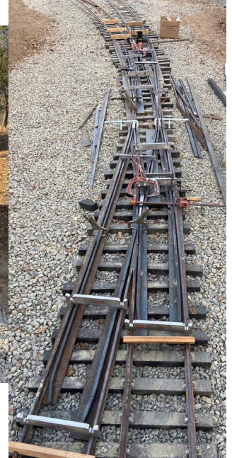
Work in progress, new loop, crossover setup, and finished welded crossover below.
