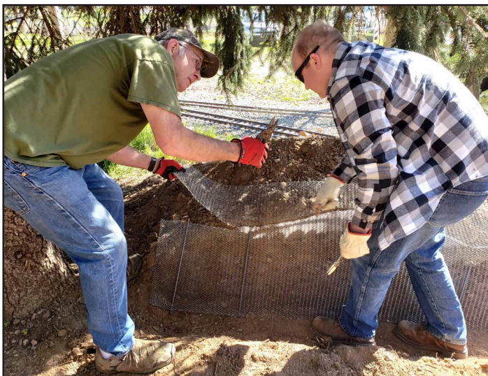
Gordon Moser and Tom Nance working on Shady Hollow retaining wall
