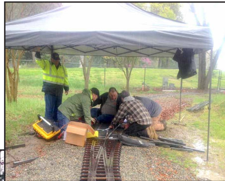
Installing the diamond thanks to a few hard working members.
