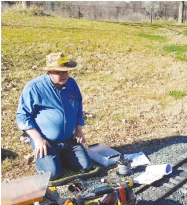
Alan Shifley - wiring signals.
