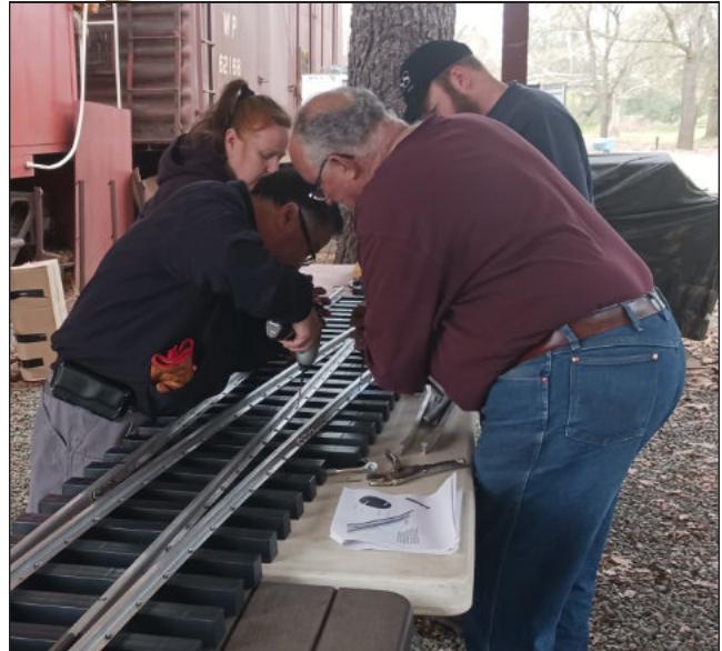
Putting new track turnout together - Steve Milward, Margaret Dobbins, Henry Nanjo, Tom Nance.
