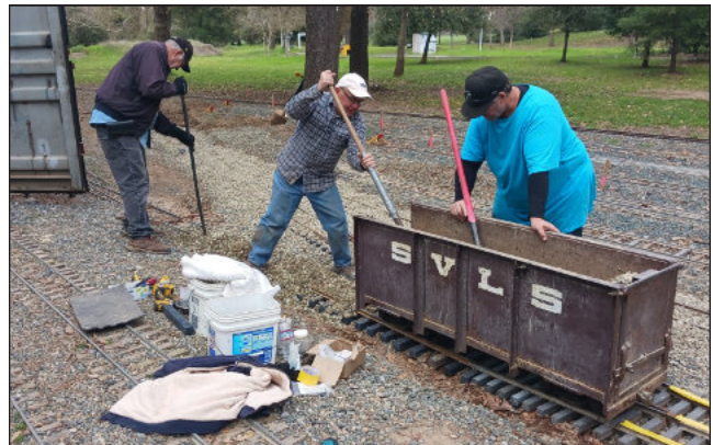
Gordon, Dave, Richard tamping ballast
