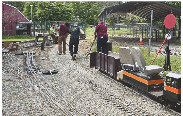
Spreading gravel for Lower Yard rebuild
